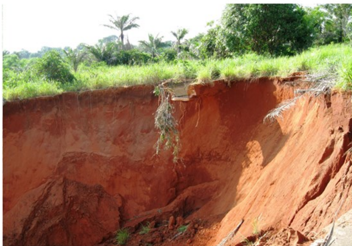
Figure 1: Typical Gully cutting in Nanka, Anambra state (Source: News agency of Nigeria, 2011)
