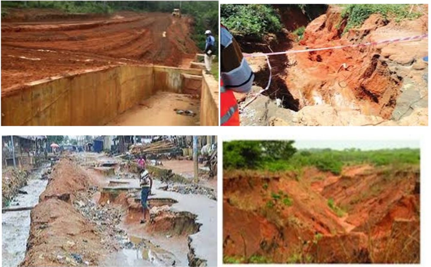
Figure 6: Typical erosion sites in Iyiuzo, Ogberuru, Ihioma and Orlu, Imo state (Source: News agency of Nigeria, 2011)
